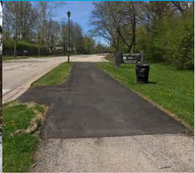
Trail extension on Trail Way
